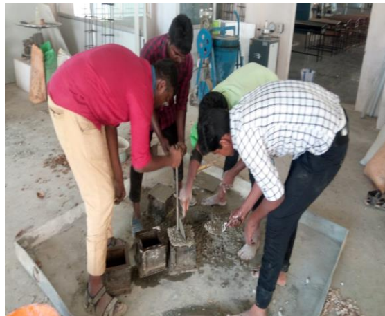
Fig No 2: Mixing of concrete
