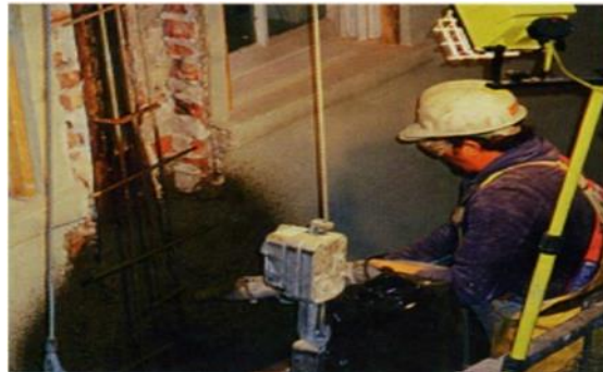
Figure 3: The application of shotcrete from a swing stage
