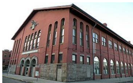
Figure 5: South Side Market House in Pittsburgh, Pennsylvania, United States.
