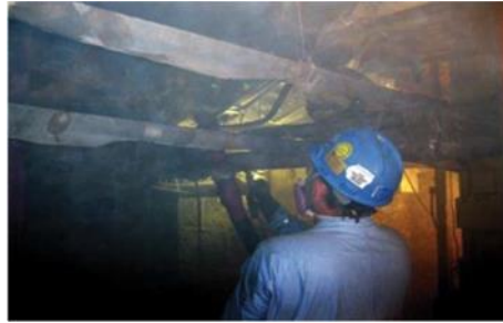
Figure 7: The application of shotcrete in an especially congested area of the basement behind the elevator shaft
