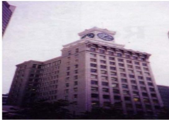
Figure 4: The north and west elevations of the Vancouver Block Building after the rehabilitation works.
