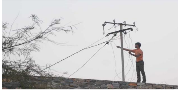
Fig[1]:Power theft in transmission lines
