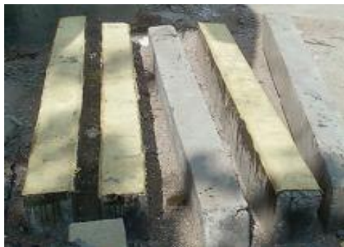
Fig 1: Casting of beam
