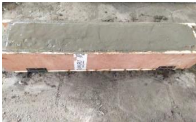
Fig 2: Epoxy - hardener and fixing of Kevlar fabric on the beam
