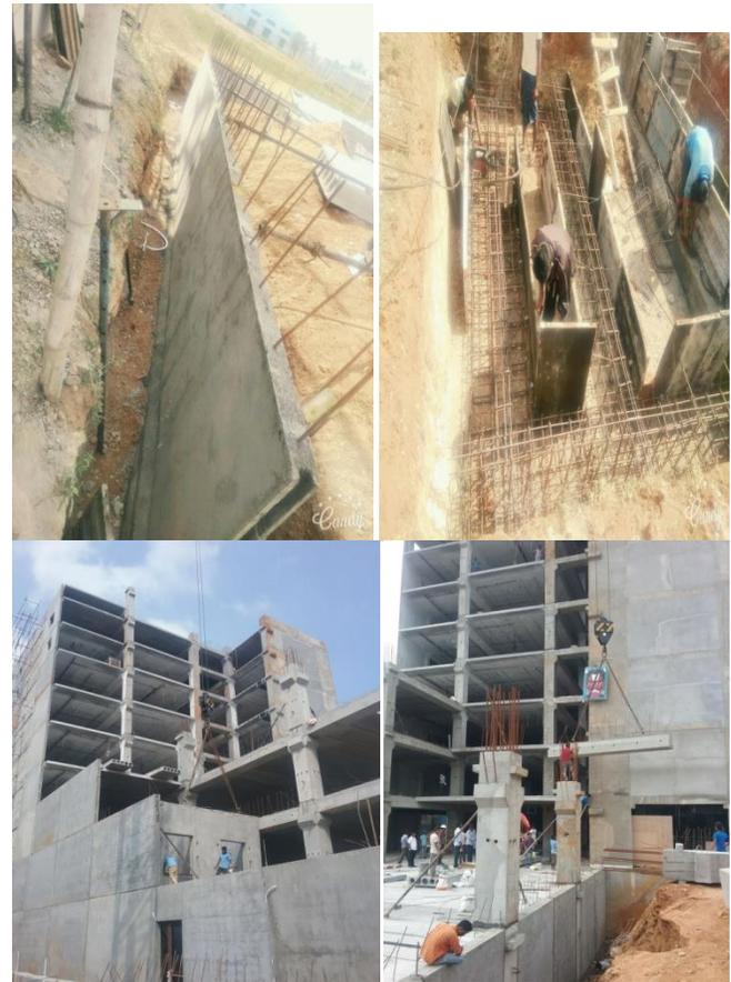
*Fig. 3.2 Precast Wall Constructions*
