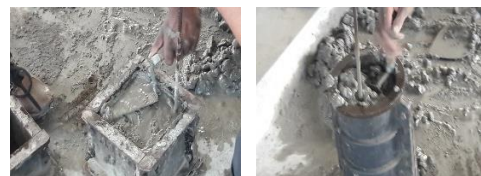
Fig 2: Casting of Cube
