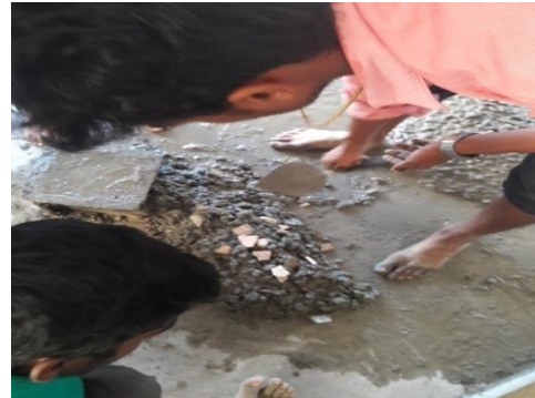
Fig No 2: Mixing of concrete
