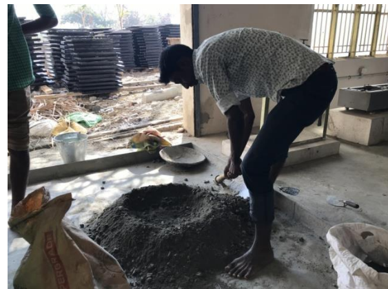
Fig No 1: Mixing of concrete
