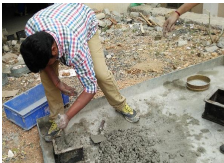
Figure 2: Mixing of concrete
