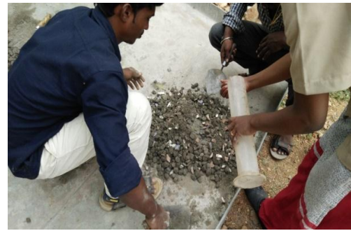
Fig No 2: Mixing of concrete
