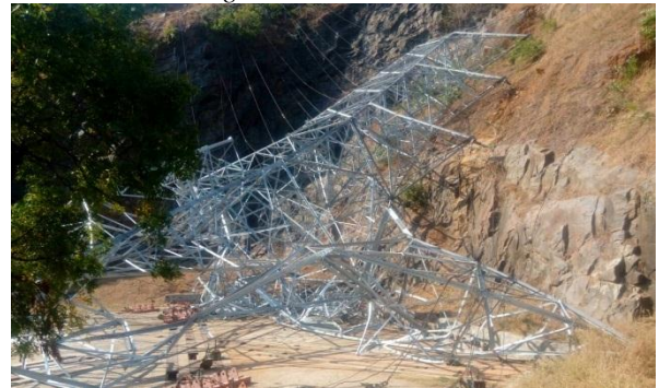
Fig 3.2.3 Failed Tower
