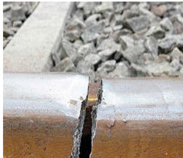
Fig1. Crack in the track
